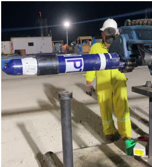
Preparing the third HSRT prior to starting the casing run.
